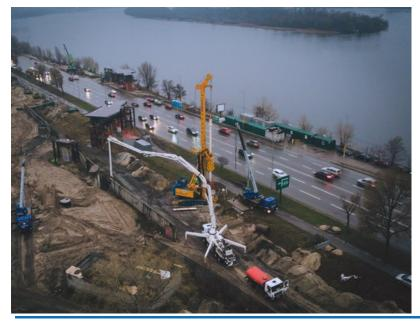
The press service of the group reported on Tuesday that a total of 55 piles with a diameter of 1.5 meters were drilled and concreted. About 2,500 cubic meters of monolithic concrete was used. To carry out these works, powerful equipment was involved – Bauer BG 45 and BG 36drilling rigs.
